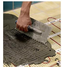
**6** Mount the new tiles on the adhesive. Joint the tiles and let the floor dry for two weeks before turning on the heating.
