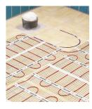
**5** Cover with one layer of flexible tile adhesive/self-levelling compound and allow it to dry before tiling or lay the adhesive and tiles in one operation. A flexible adhesive and grout should always be used.
