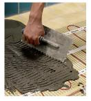
6 Mount the new tiles on the adhesive. Joint the tiles and let the floor dry for two weeks before turning on the heating.
